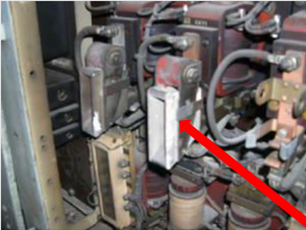
Switch gear flash guard and electrical wiring
